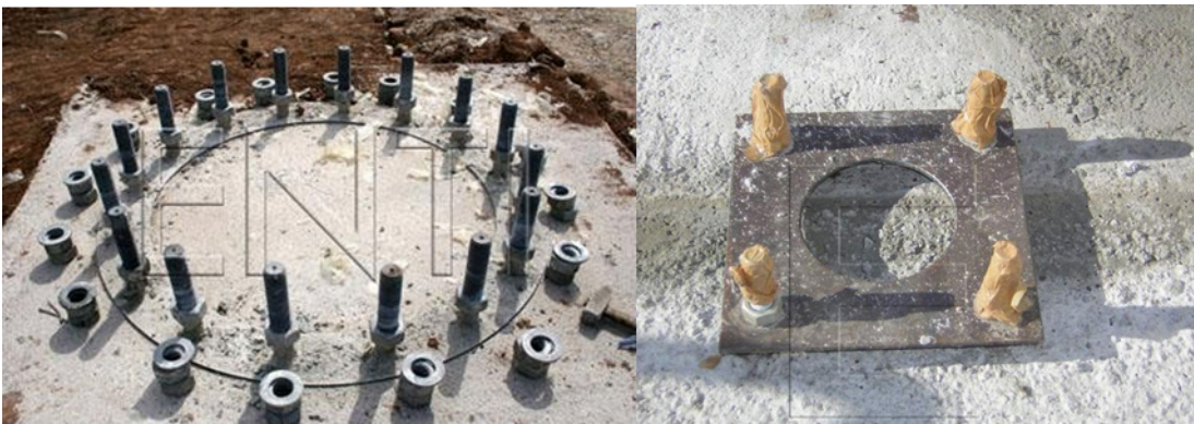
Picture 1.1: Various anchor bars
