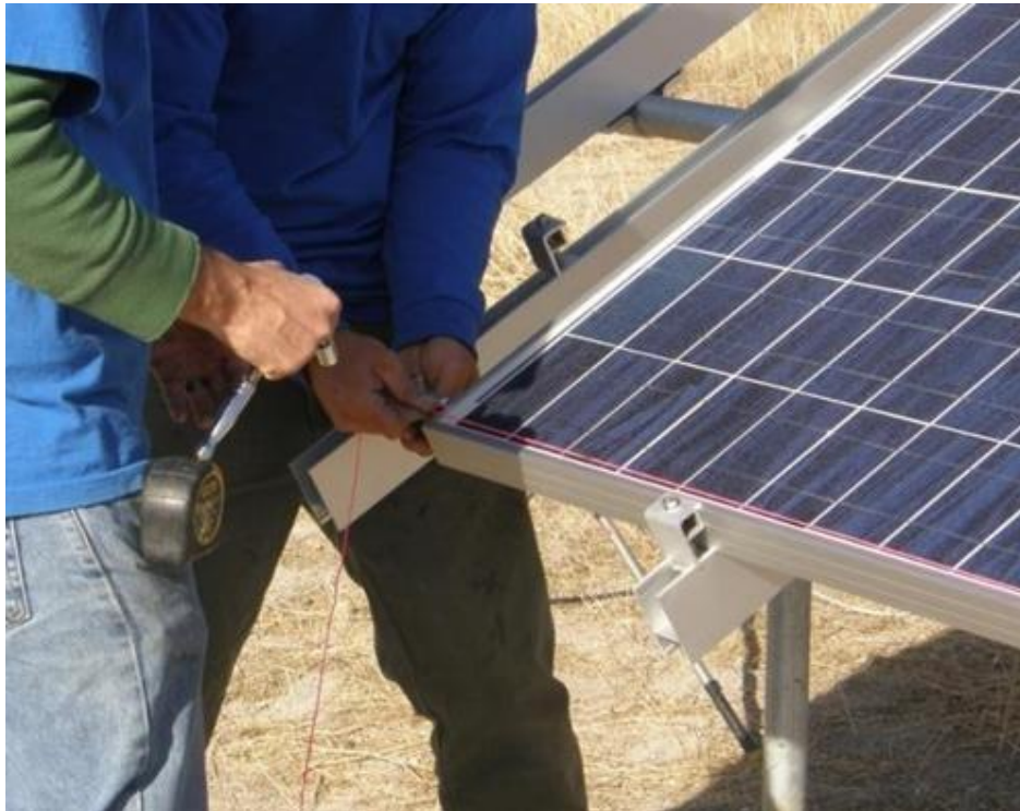
Picture 4.1: Keeping solar panels aligned while arranging them
