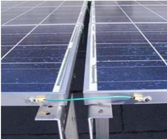
Resim 2.2:a) Use of wrong lug and wire
