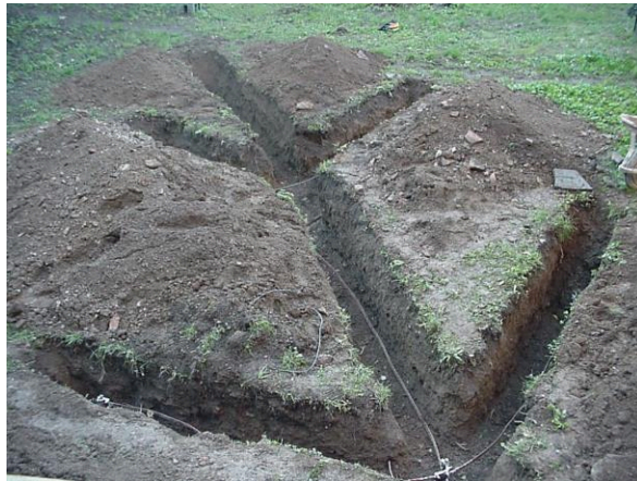
Figure 2.2: Crow's foot grounding system
