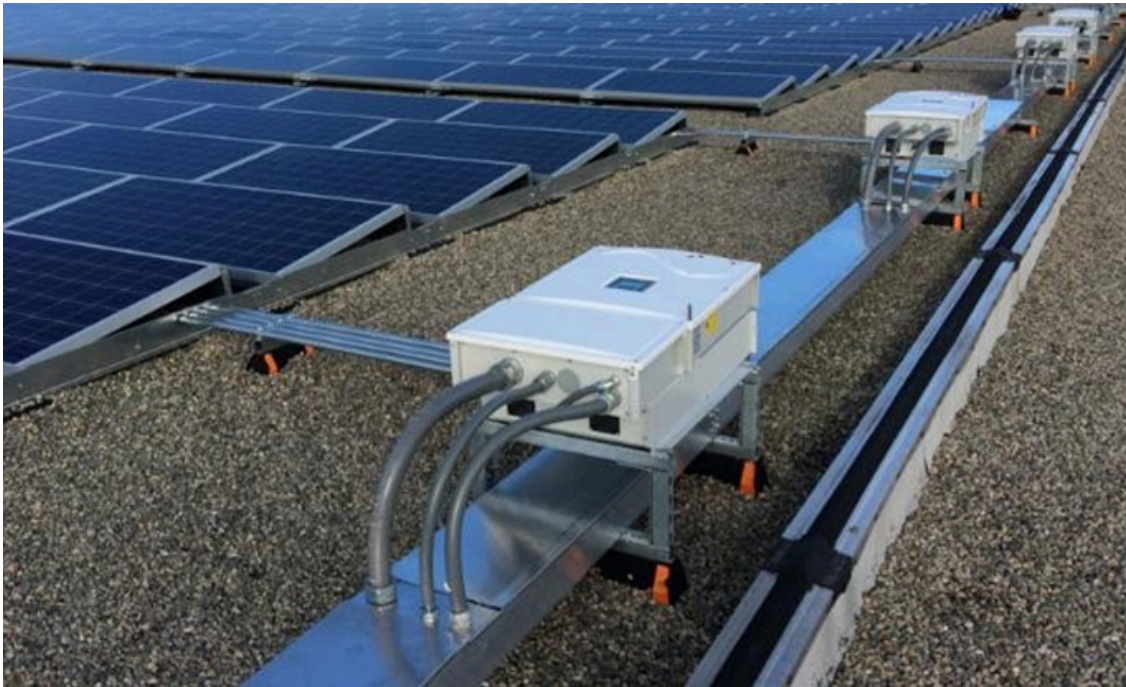
Picture 2.1: Cable installation between panels
