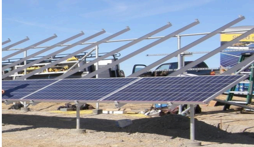
Picture 4.2: Solar panels laid on profiles
