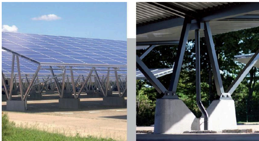
Picture 1.6: Metal carrier concrete shapes where solar panels are mounted
