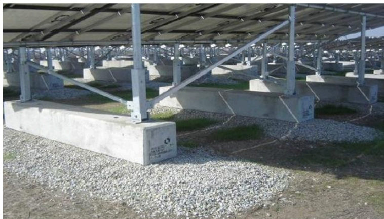
Picture 1.4: Metal bearing concrete and anchors balanced on a scale in the solar power plant
