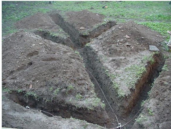
Figure 2.2: Crow's foot grounding system
