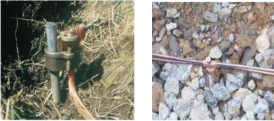
Picture 2.3: Connecting the grounding conductor to the grounding rod
