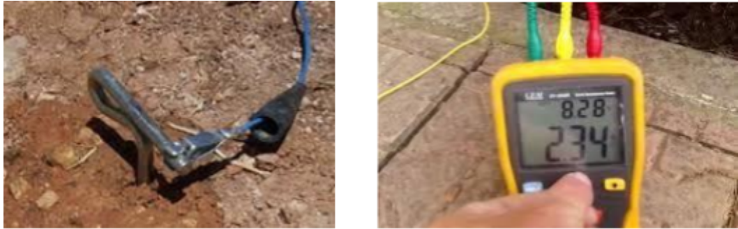
Photo 1.6: Meger pile connection and resistance measurement
