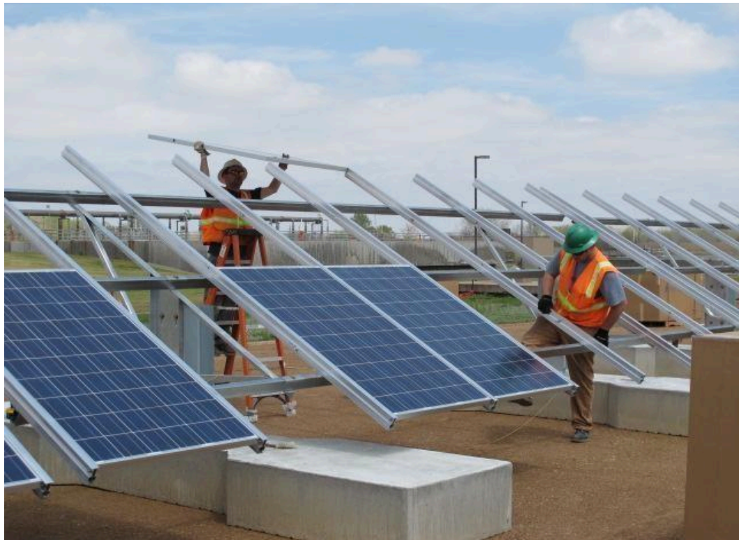
Picture 1.2: Solar stand installation
