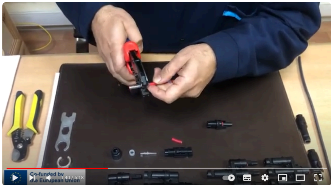
Picture 3.7: Solar connector connection
