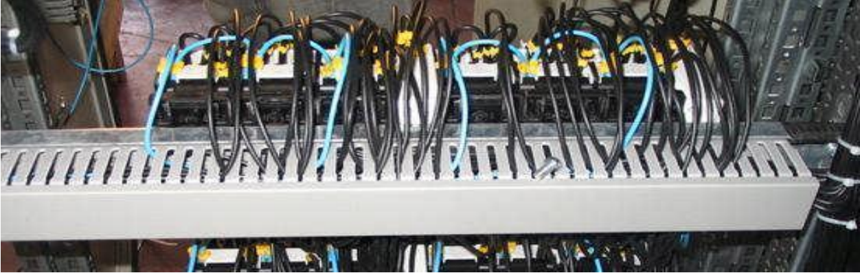
Picture 2.8: Cables completed in duct placement
