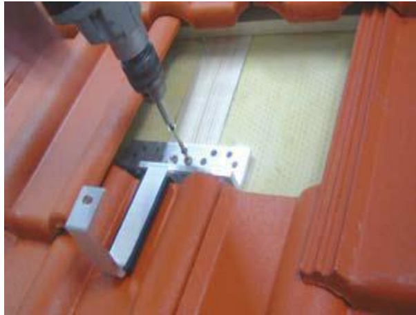
Picture 2.5: Installation of roof brackets on beams
