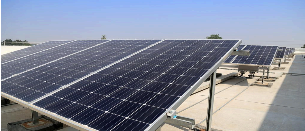
Picture 1.2: Panel installation on a flat roof
