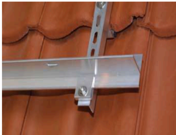
Picture 2.5: Installation of roof brackets on beams
